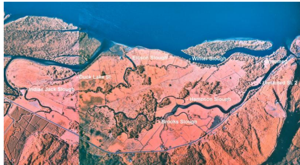
Suite of Tide Gate Replacement Actions Courtesy of U.S. Army Corps of Engineers
