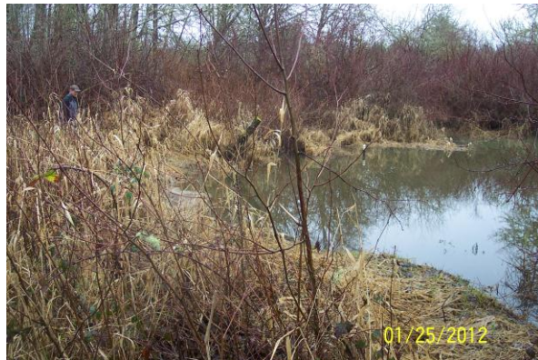
Site Photo 6: South end abandoned logging road culvert and fill.
