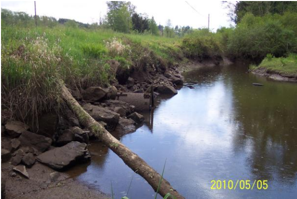
Site Photo 1: Outlet and tide gate at SR-4 MP 34.09.
