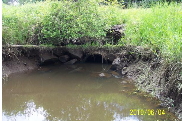
Site Photo 2: Inlet culvert and tide gate at SR-4 MP 34.09.
