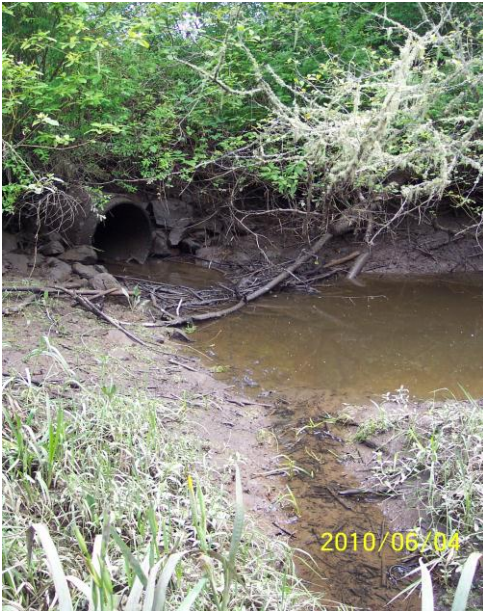
Site Photo 3: Outlet of culvert at SR-4 MP 33.94
