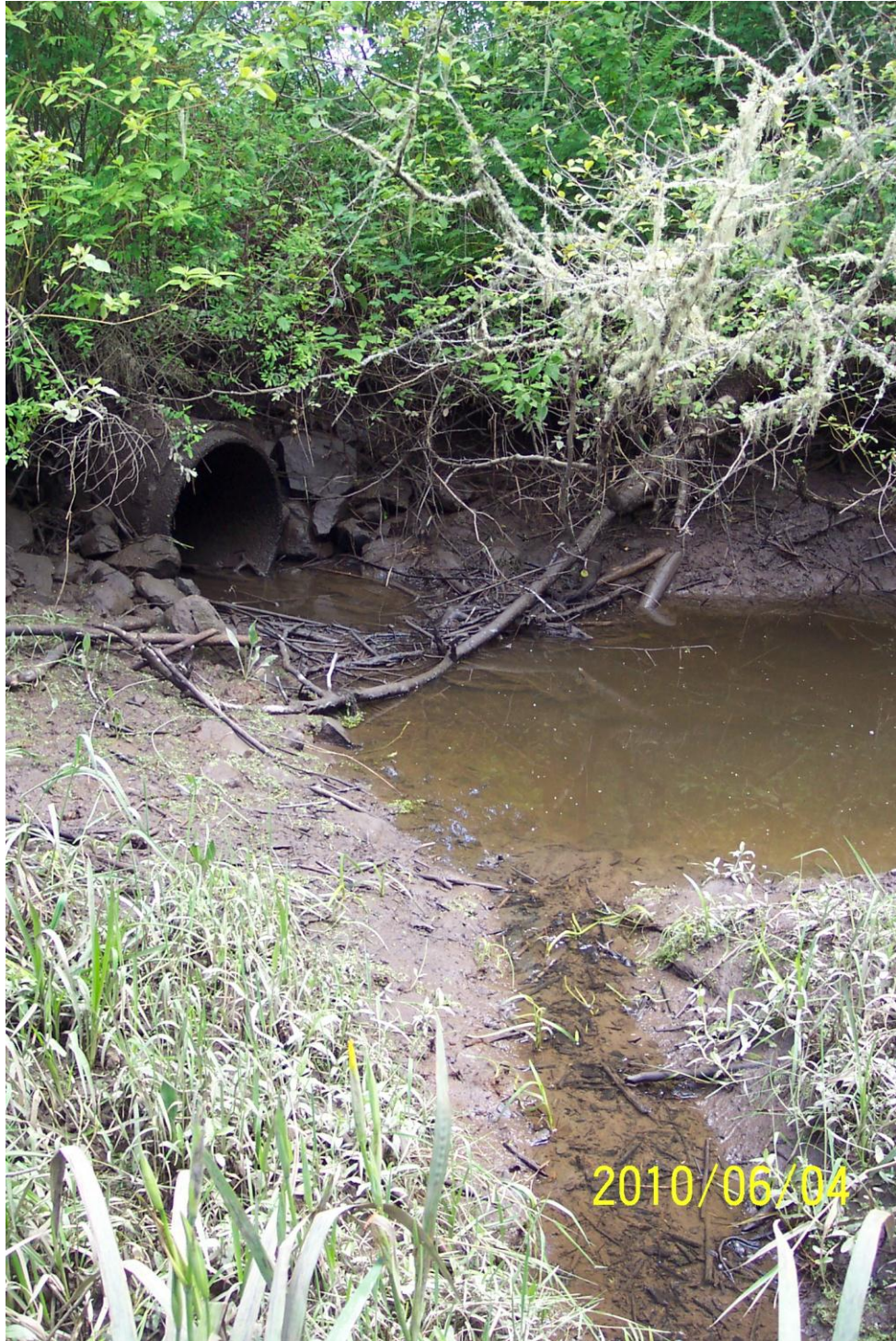
Figure 9. West (Elochoman Slough) end of culvert at MP 33.94 Hwy 4.
