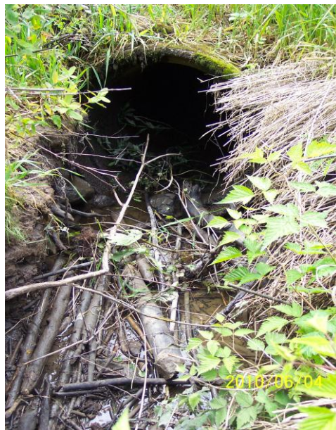
Site Photo 4: Inlet culvert at SR-4 MP 33.94.
